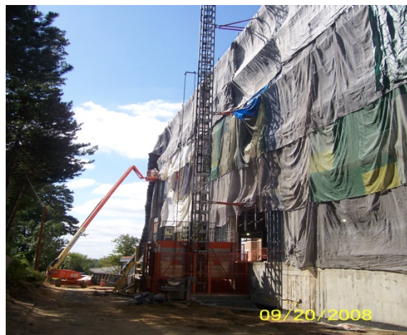
FIGURE 2- EAST ELEVATION WITH MATERIAL HOIST IN PLACE
