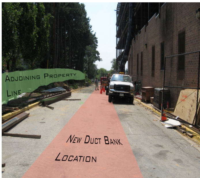
FIGURE 1- VIEW LOOKING FROM THE NORTH TO SOUTH OF THE ONLY ACCESS ROAD ON SITE
